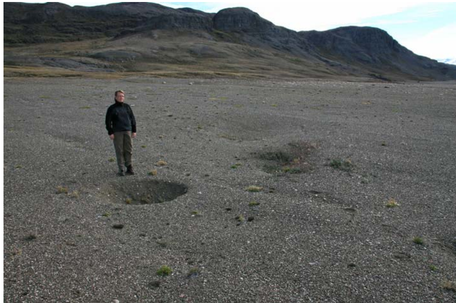
Figure 19. The subsided sump at the Gro#3 drill site on Nuussuaq Peninsula in 2007. The sump was established in 1996 in the flare pit close to the well and was used for the solid fraction of the drilling mud. The drill site is a natural gravel bank.
