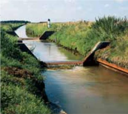
The channelisation of Danish streams increased the slope of new straightened stretches. Trapezoid weir-like constructions were built in many streams, to dissipate energy from the increased slope over short segments of the stream. Unfortunately these constructions also act as obstructions limiting the free migration of fish and macroinvertebrates. Today many of these obstacles have been transformed into riffles by local water authorities.
