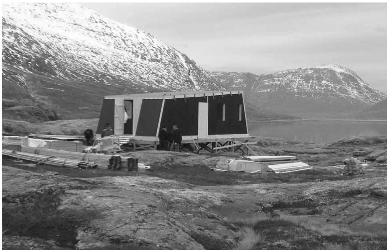
Figure 1.2 Topping-out ceremony for the new research hut at Kobbefjord, October 2008. Photo: Søren Rysgaard.
