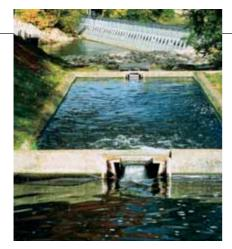
A fish guidance fence and fish ladder at the Tange Hydropower Dam on the River Gudenå.
