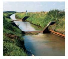
The channelisation of Danish streams increased the slope of new straightened stretches. Trapezoid weir-like constructions were built in many streams, to dissipate energy from the increased slope over short segments of the stream. Unfortunately these constructions also act as obstructions limiting the free migration of fish and macroinvertebrates. Today many of these obstacles have been transformed into riffles by local water authorities.
